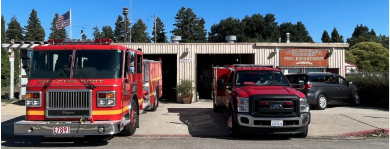
The current Santa Margarita Fire Station
